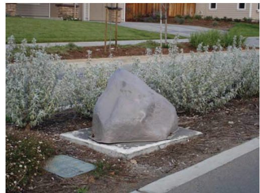
Landscape/Irrigation equipment should be screened or covered. Fake boulder shown.
