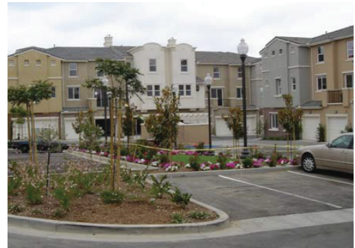
Parking area located behind the building away from the street.
