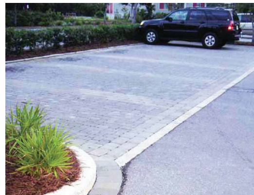
Permeable pavers at parking spaces
