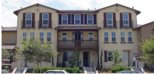
Multi-family residential projects should use varied roof forms to prevent a box-like appearance.
