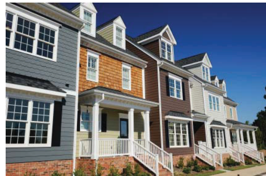
The utilization of dormers on the third story helps to improve the street level scale of the building.
