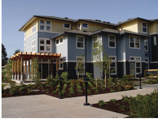
Heavier and darker colors should be used at the base of the building.
