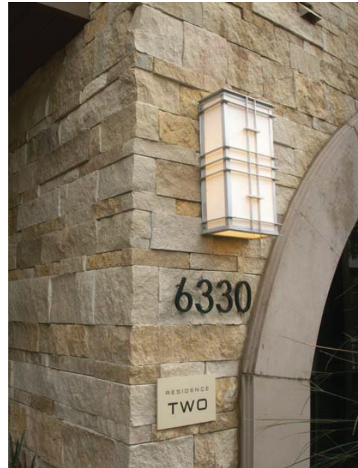
Light fixtures should be selected to be architecturally compatible with the main structure.
